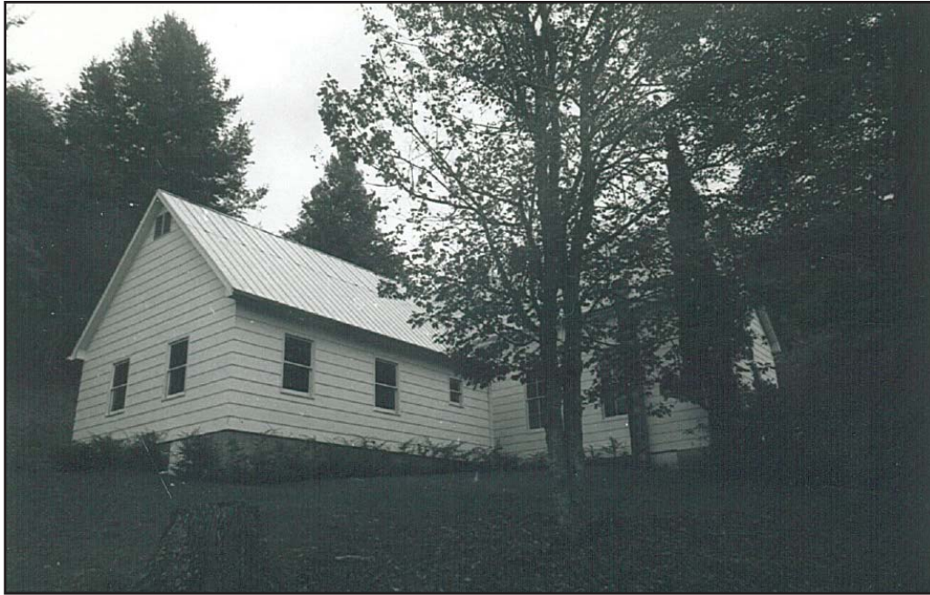
Photograph 7: Northeast elevations of the church and addition and the northwest elevation of the addition; looking southeast. (Source: 1989 Historic Sites Survey)
