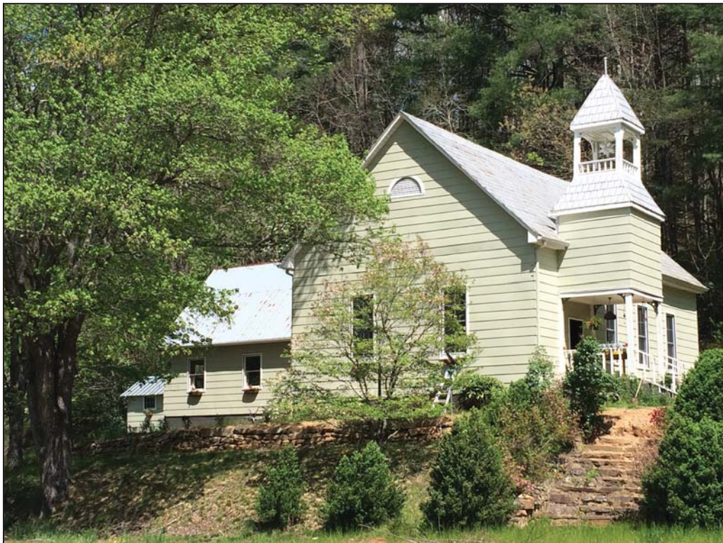
Photograph 6: Southwest and northwest elevation of the church; looking northeast. (2016)
