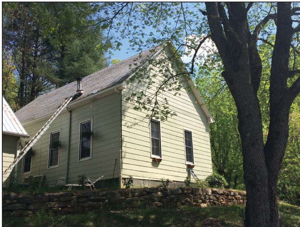
Photograph 10: Northwest and northeast elevations of the church; looking southeast. (2016)
